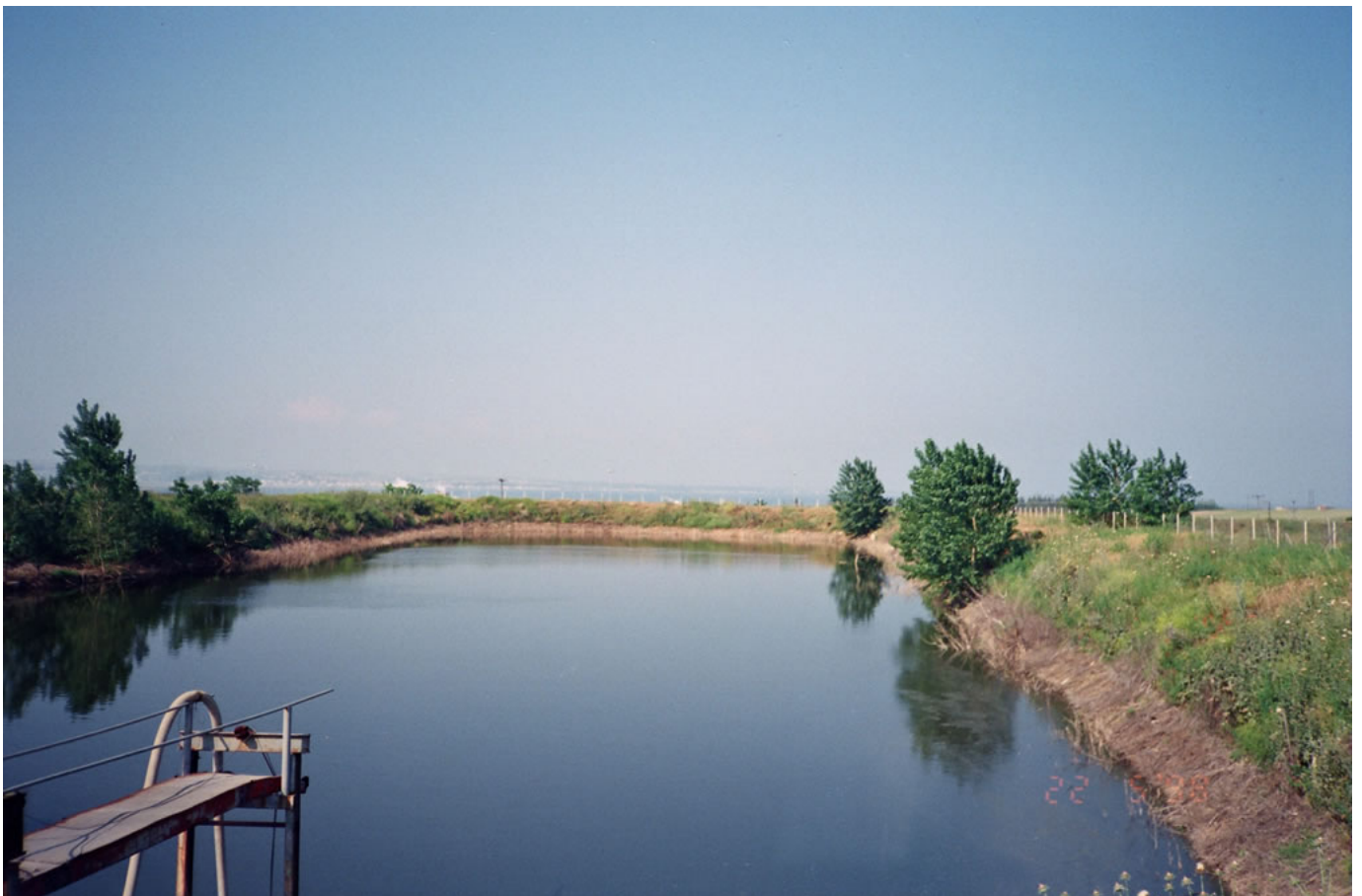
Condition May 1998 after less than 1 year of PLOCHER treatment
